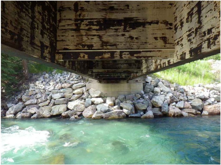
RIGHT BANK ABUTMENT
